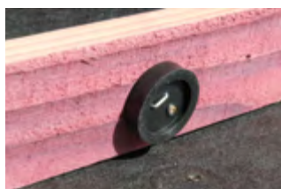
Standard Battens block water flow
