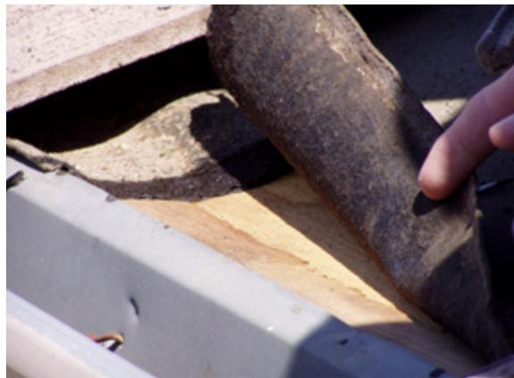
The other problem with the raised fascia method is that it eliminates the option of using proper eave riser metals, including those designed for improved ventilation. In an era where ventilated tile roofs are being touted as effective energy-saving assemblies, the air intake at the eave is severely limited or even totally eliminated by the fascia board.
