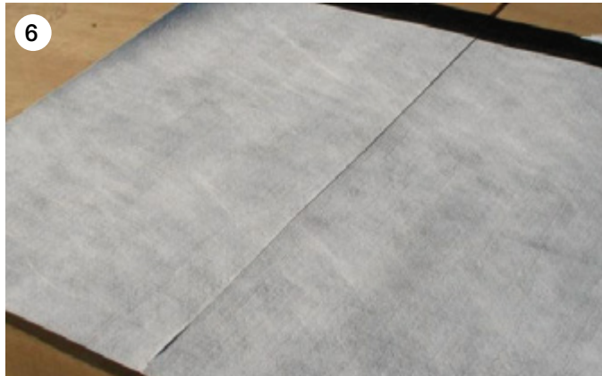
Completed Inverted Sheet Seam (Pic. 6)
